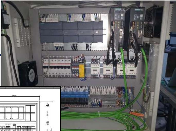
Electrical Control System with Siemens S7-1200 PLC and V90 PN series Servo for Motion Application.
